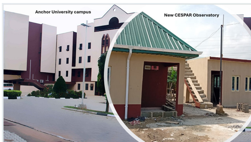
Figure 2. CESPAR mini-observatory facility (at final stage of completion) at Anchor University, Lagos, Nigeria. Inspired by the success of the SCOSTEP/PRESTO-supported magnetometer database project, the observatory was approved by the university to provide dedicated infrastructure for ground-based solar-terrestrial observations, data archiving, research activities and capacity building in space science and technology.
