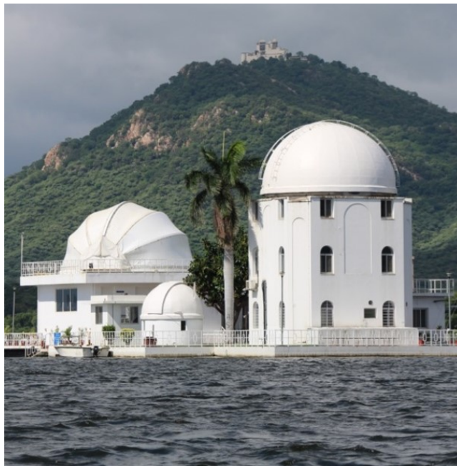
Figure 1. The housing and the dome (left) for MAST on the island observatory in the lake Fatehsagar of Udaipur.
